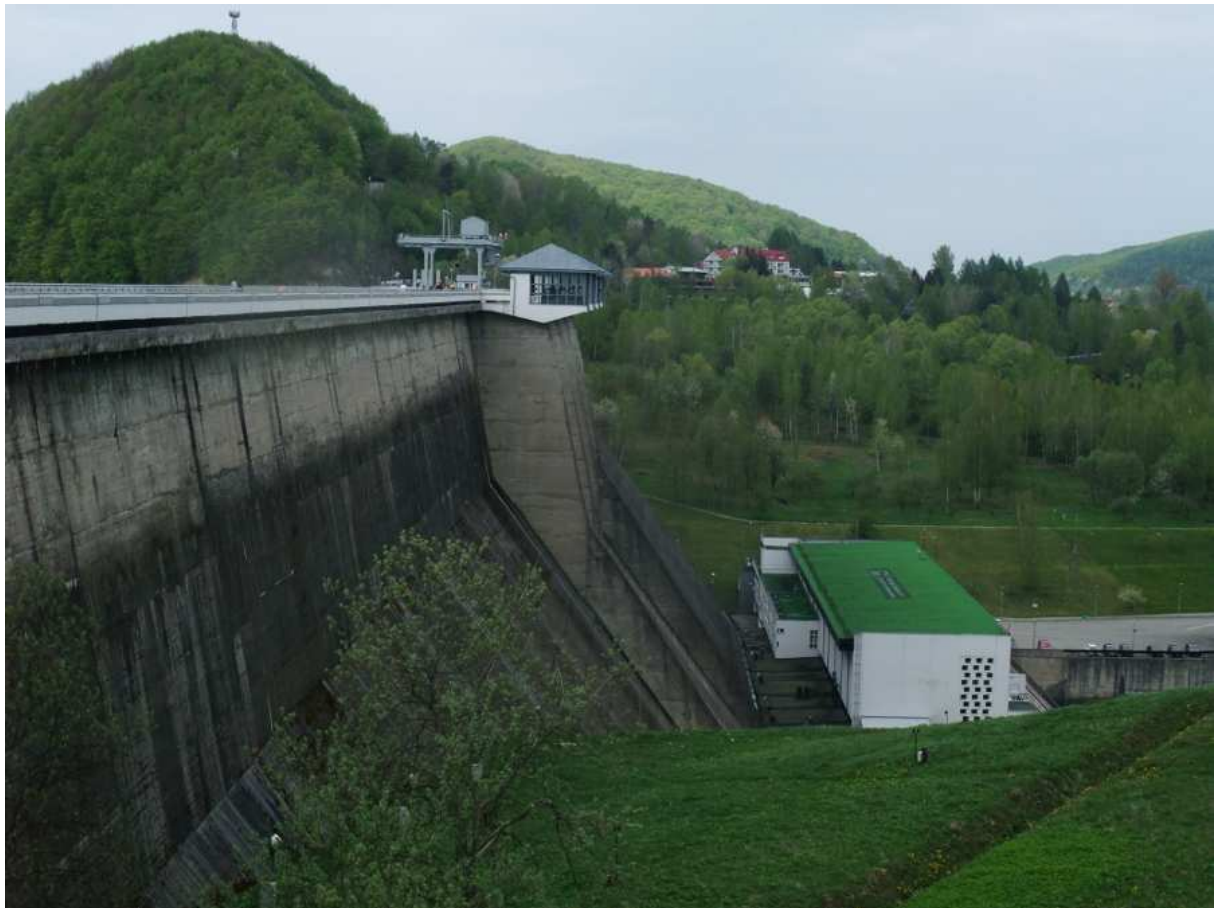
Fig.40 A concrete dam in Solina, Poland. Source: own work.
