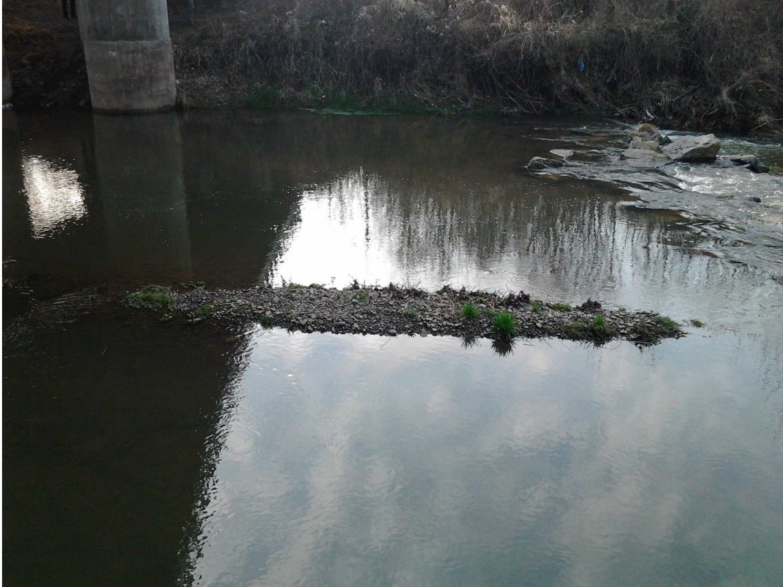
Fig.24 A pile of gravel stored behind a pillar of a bridge. Source: own work.
