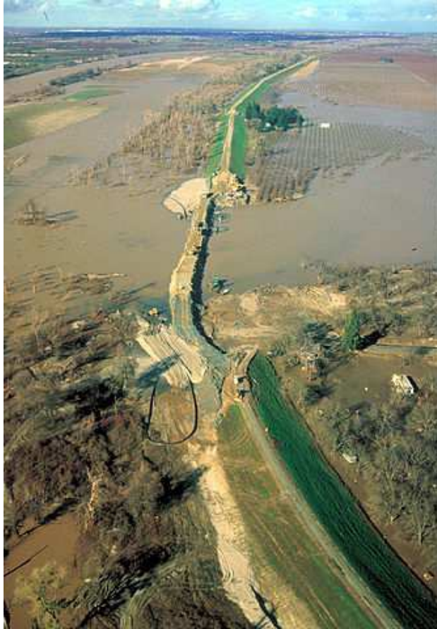
Fig.34 A broken levee by Sacramento river, USA. Source: Wikipedia [W9].
