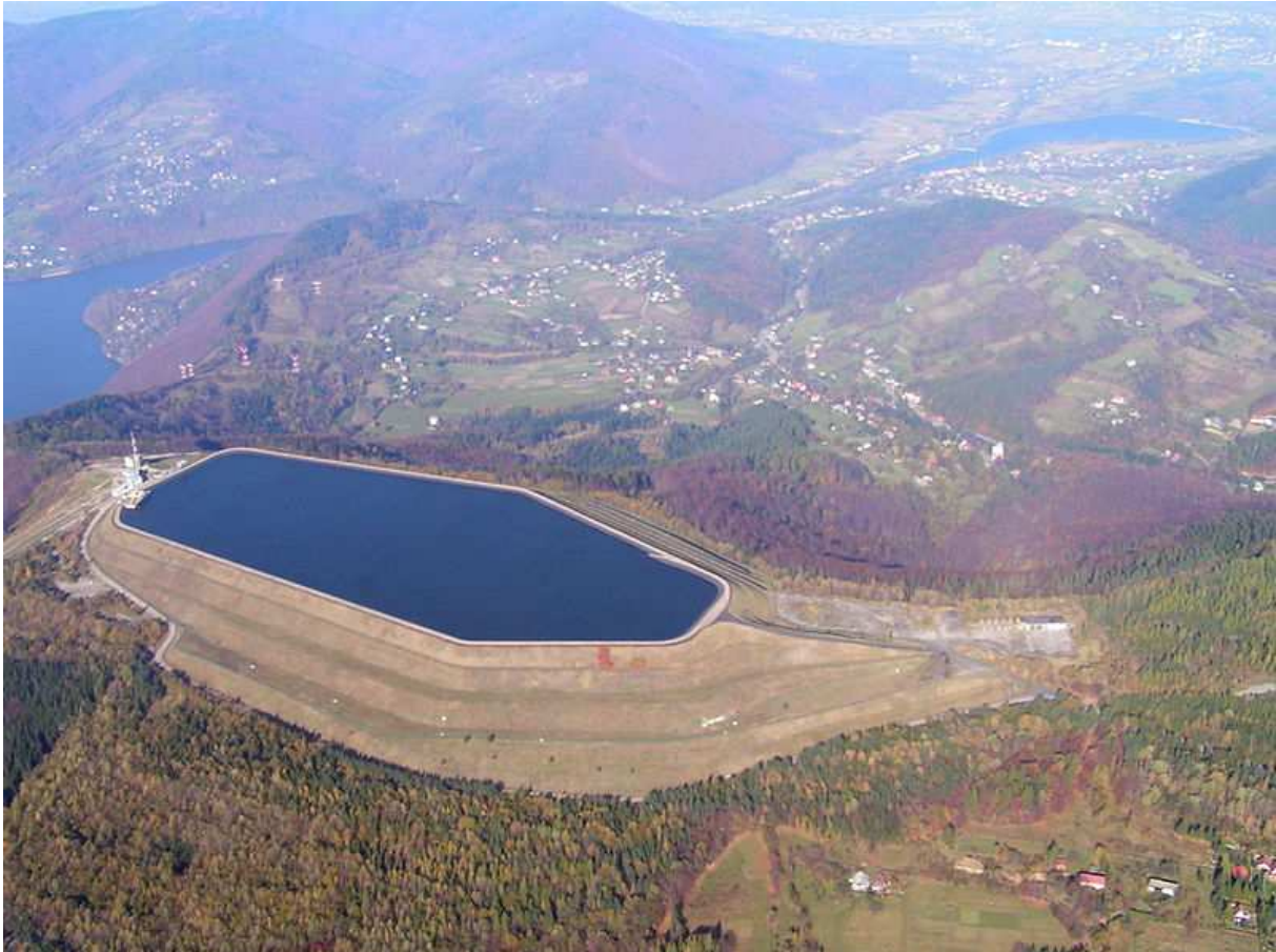
Fig.46 Pumped-storage power plant in Porąbka-Żar, Poland. Upper reservoir on the top of a mountain, the lower reservoir visible in the background. Author: Ongrys. Source: Wikipedia [W13].
