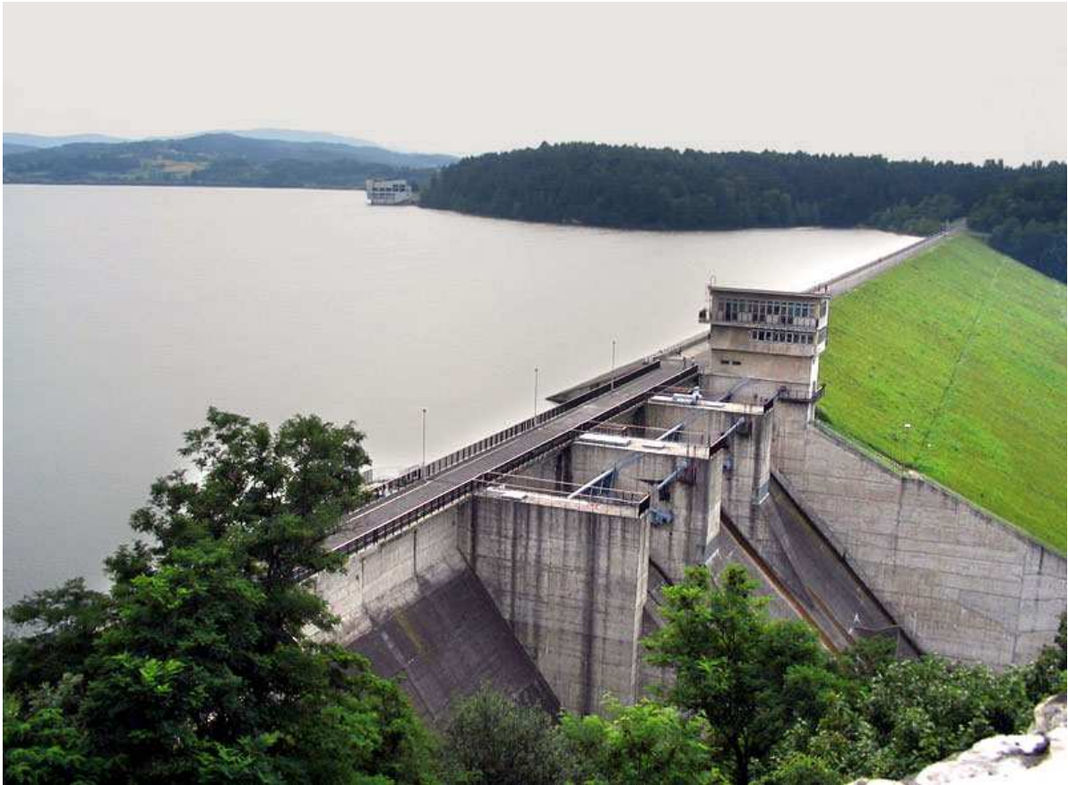
Fig.39 Dobczyce Lake, Poland – an artificial reservoir closed by an earthen dam. Created as a drinking water supply for Kraków. Source: Wikipedia [W10].
