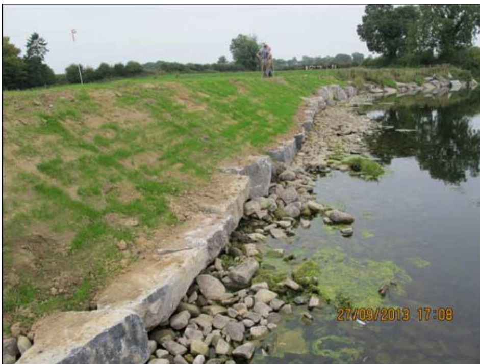
Fig.35 Bank protection on River Dinin, Ireland. Source: Inland Fisheries Ireland [E3].
