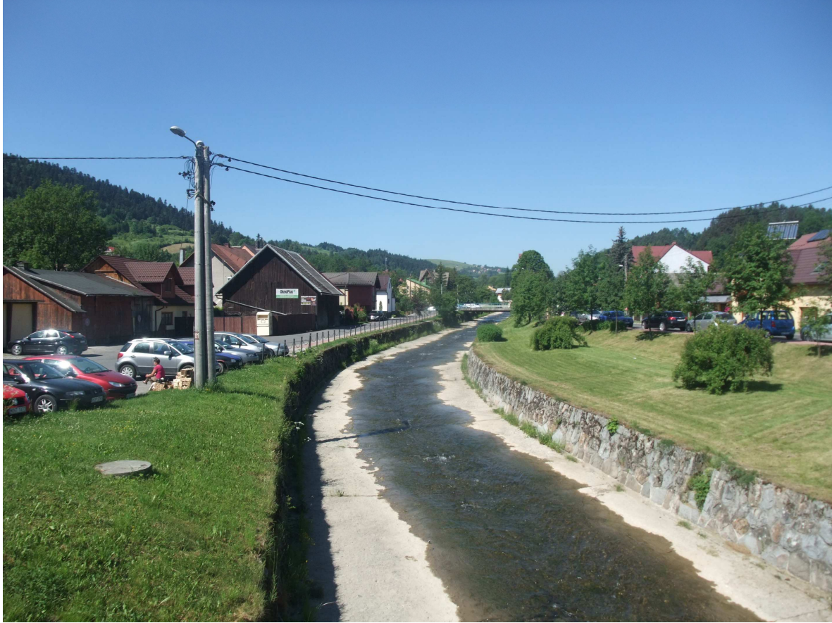
Fig.37 Heavy embankments in Krościenko nad Dunajcem, Poland. Source: own work.
